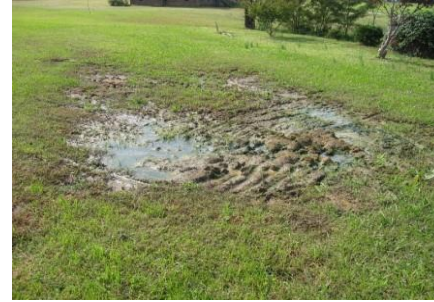
Septic system failure
