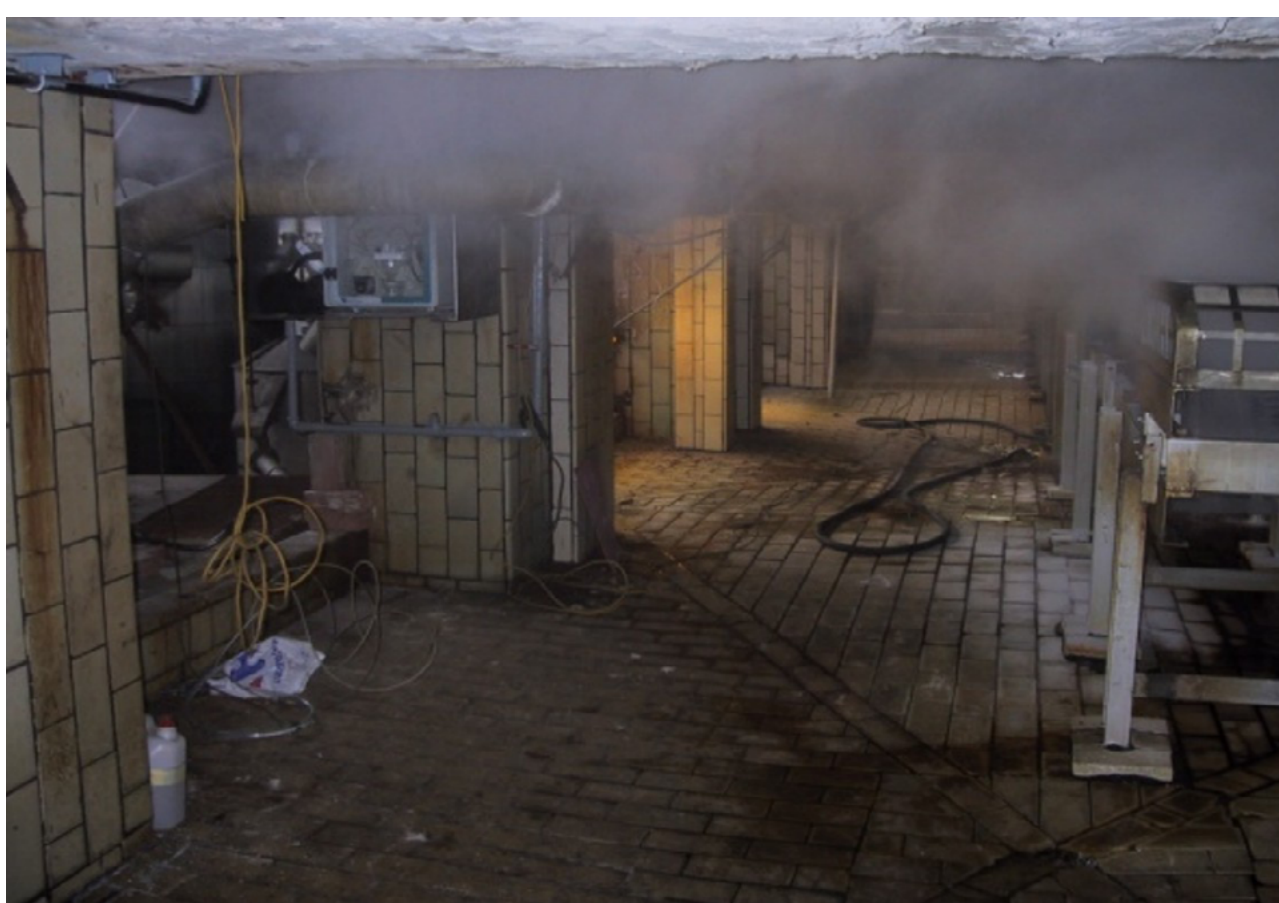
Fig. 2: Analyzer installed in a harsh, low-visibility environment with poor access and high humidity. These conditions increase maintenance burden and risk of failure.
