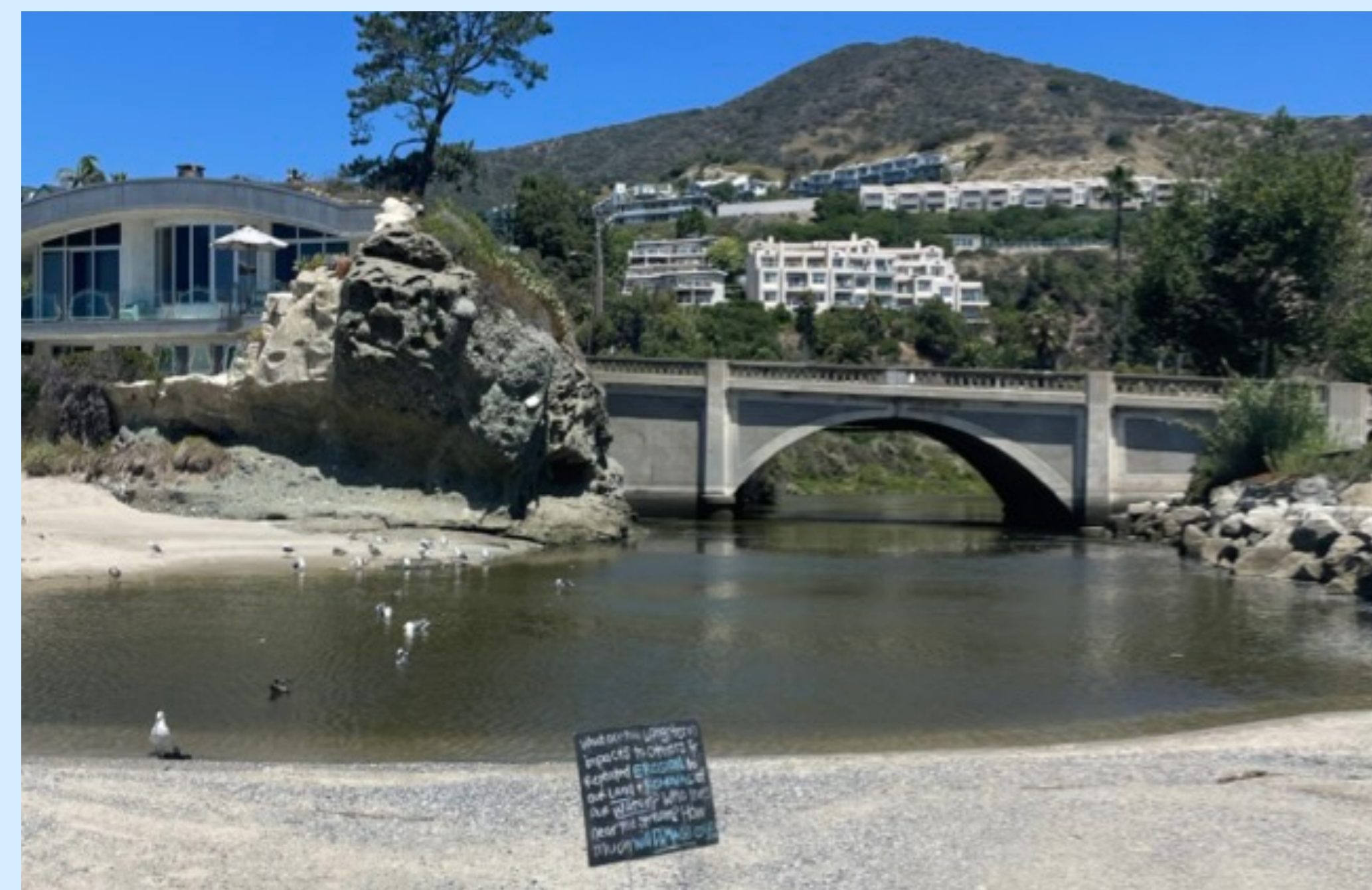
Figure 4: Aliso Creek and the Sand Berm
